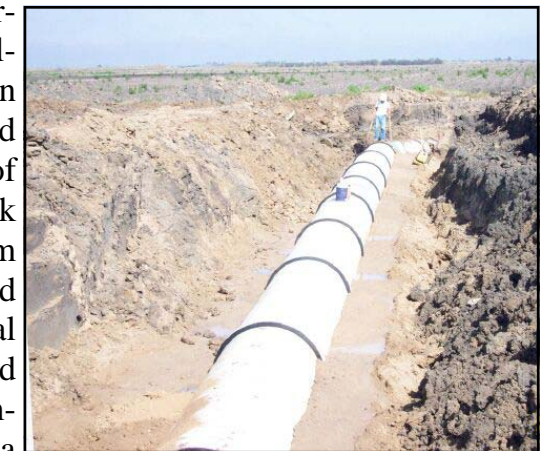
36" PVC pipe installation
