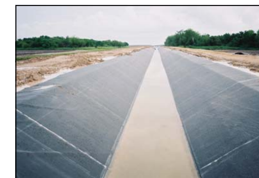
Firestone liner installation
