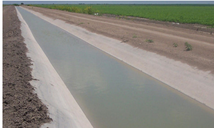
Firestone Pond Guard® Canal Liner used on the Wyrick Canal
