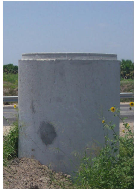
Irrigation Standpipe Used to Test Pipelines for Leaks
