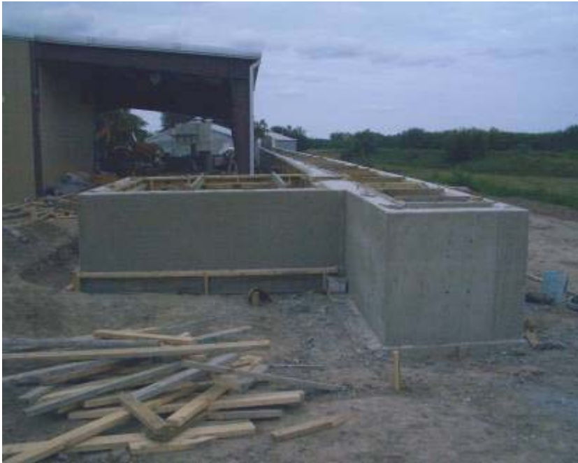
Calibration tank poured wall and flume end.
