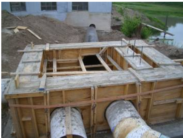
Diversion Box Foundation
